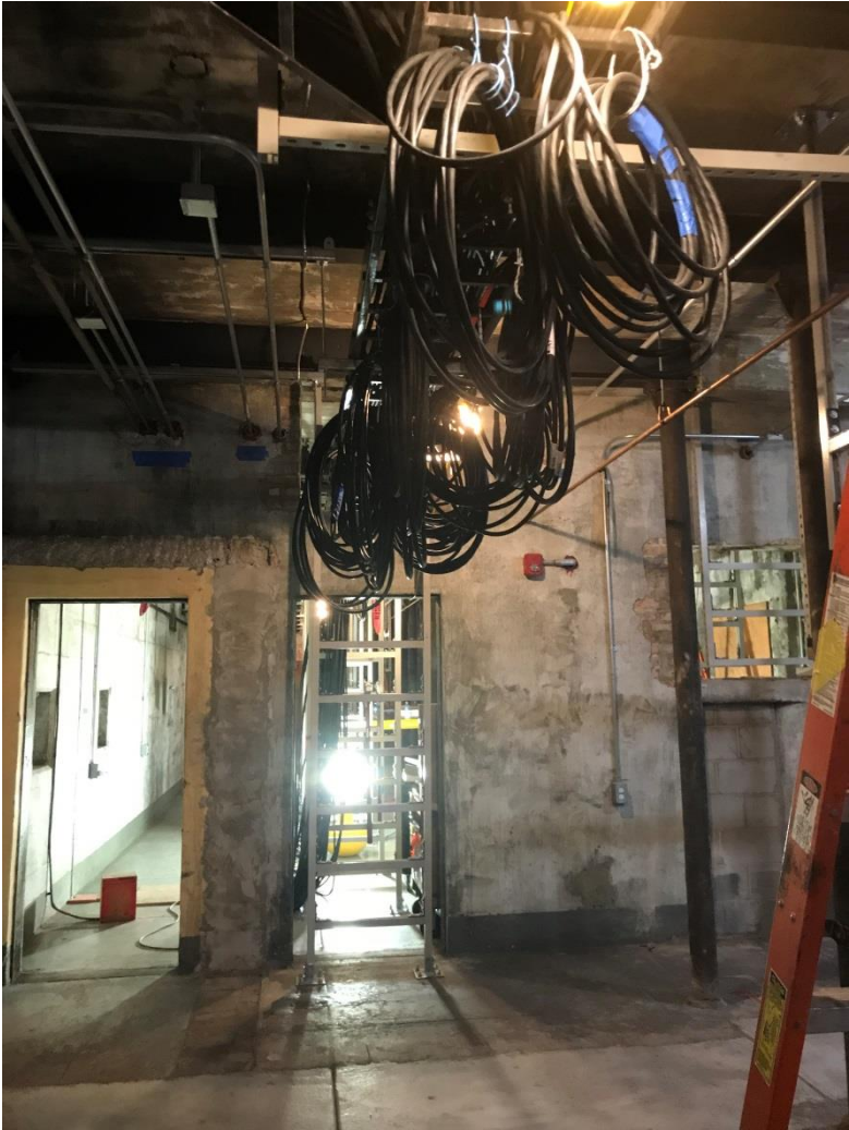
Cable Installation and Auxiliary Transformer Installation at Illinois Substation
