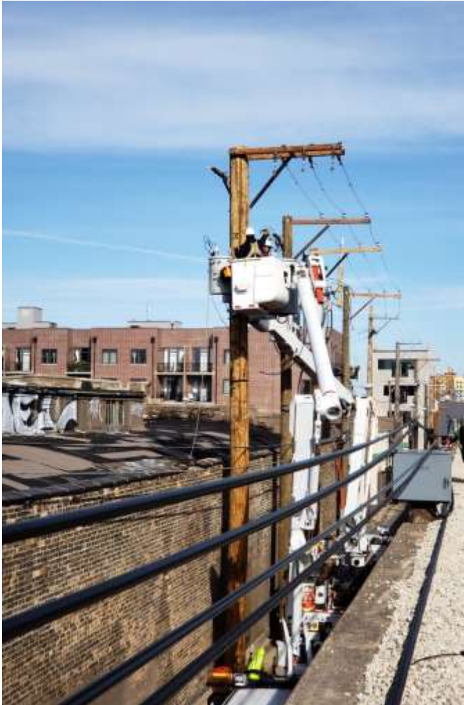
Transformer Hookup in Alley South of Winona (left) and Conduit Installation in Alley South of Berwyn (right)
