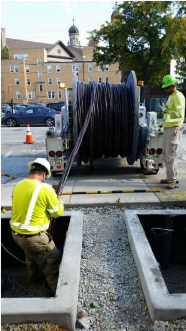
ComEd Installing Cable at Milwaukee Substation
