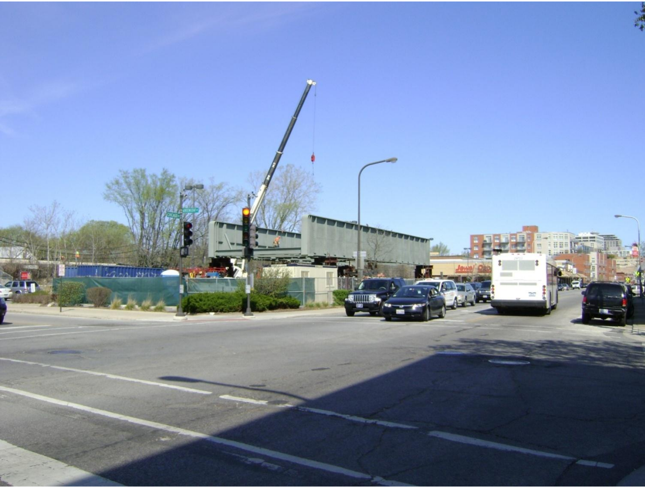
Construction of Greenleaf Bridge Span in Staging Area
