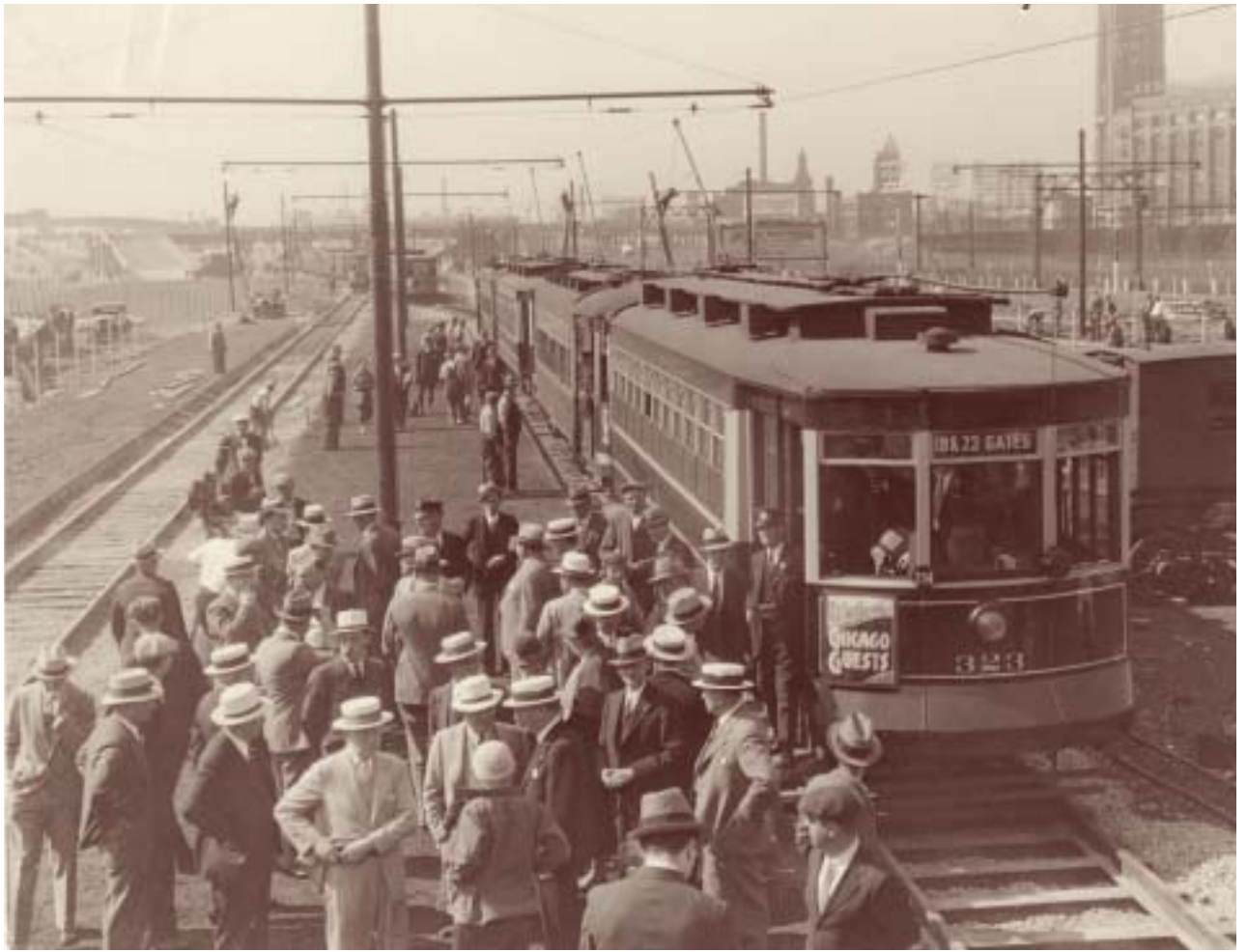
Service to the lakefront site of the Century of Progress World's Fair in 1933-34 involved extending streetcar lines over Illinois Central Railroad tracks at both Roosevelt Road and 23rd Street. In this view looking south, "Old Pullman" Car #323 has just delivered special guests to a new terminal near the south end of Soldier Field. The service ran east from Wabash on Cermak, which had recently been renamed from 22nd Street to honor Mayor Anton Cermak, and then via Silverton Way, the 23rd Street viaduct and a private right-of-way to the terminal.
