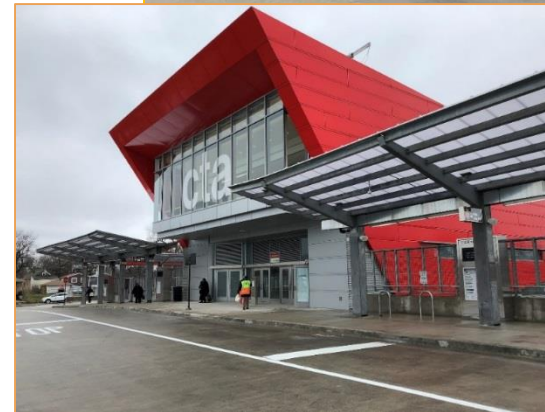
CTA Red Line 95 th Street Station
