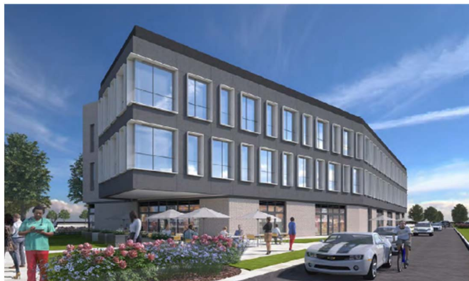
Ogden Commons Office Building – North Lawndale
