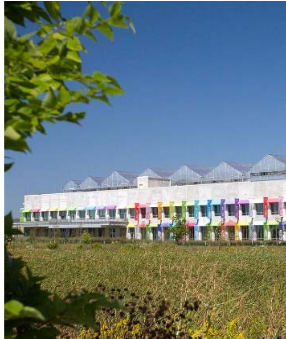
Method Factory – Pullman Industrial Corridor
