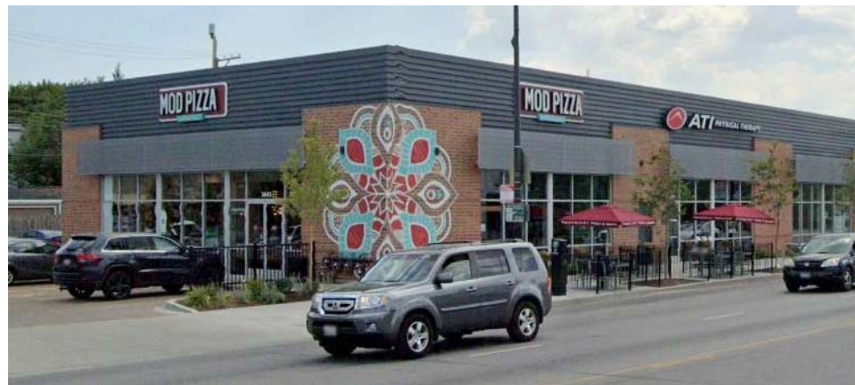
Stand Alone Retail Building – Western Avenue
