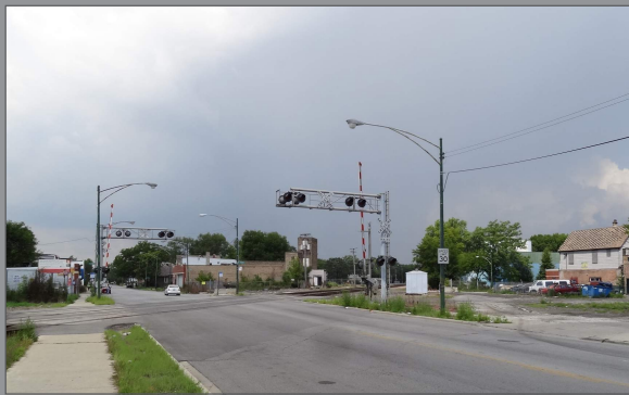
Existing - 115th Street and UPRR Tracks
