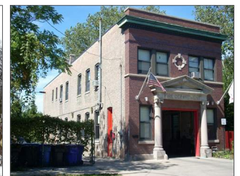
10227 S. Halsted Street (Former Classic Revival Substation)
