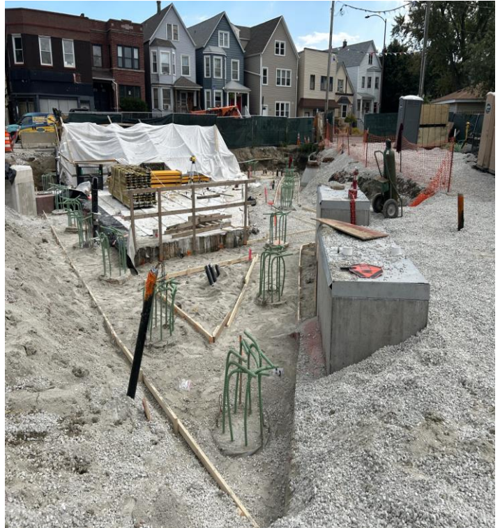
Ductbank Installation and Site Backfill at Barry
