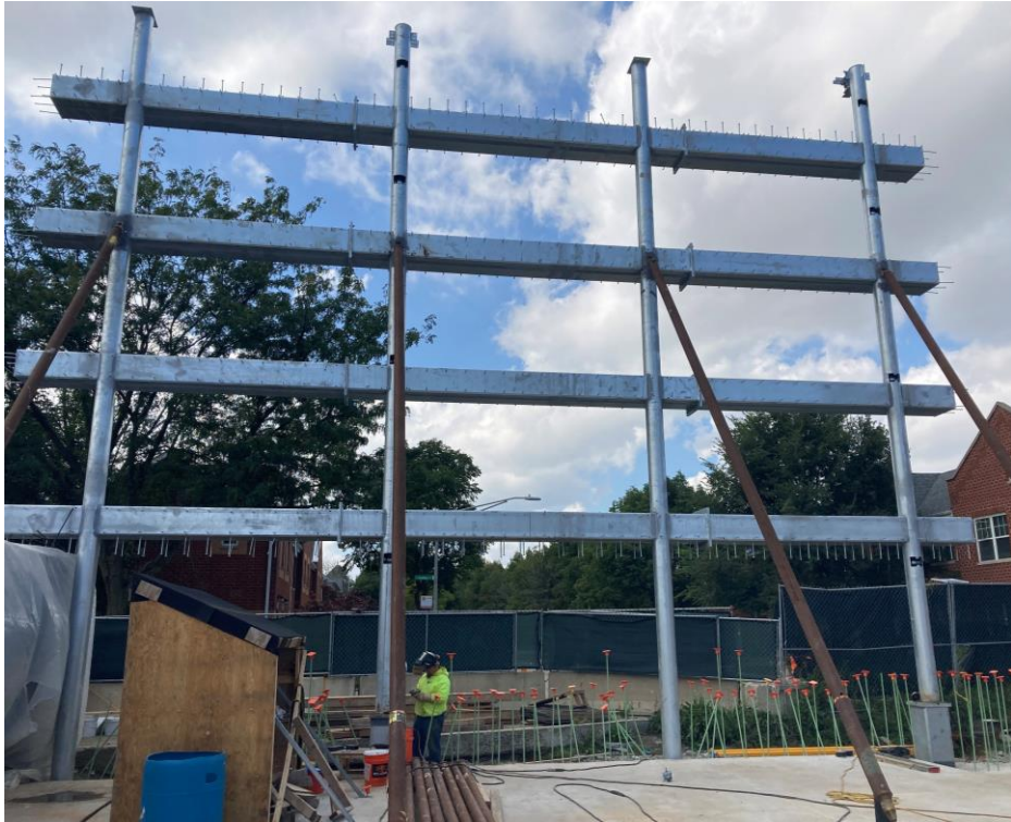
Station House Steel at West Wall
