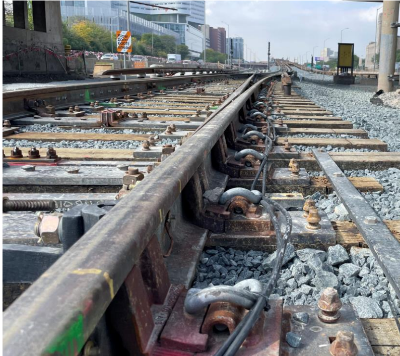
Trackwork complete at Loomis
