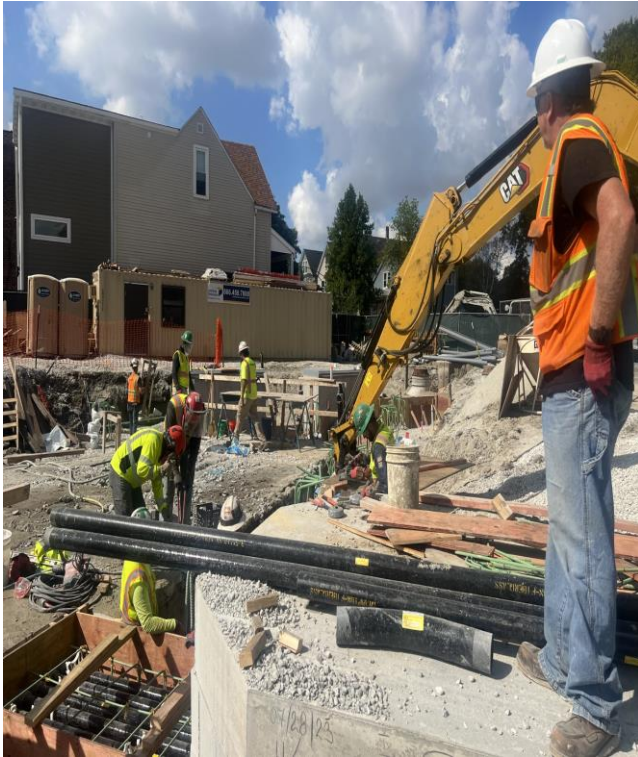
Ductbank Installation and Site Backfill at Barry
