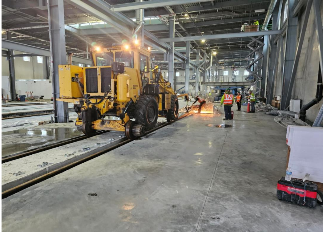
Installing Rail at Track D – Facing North
