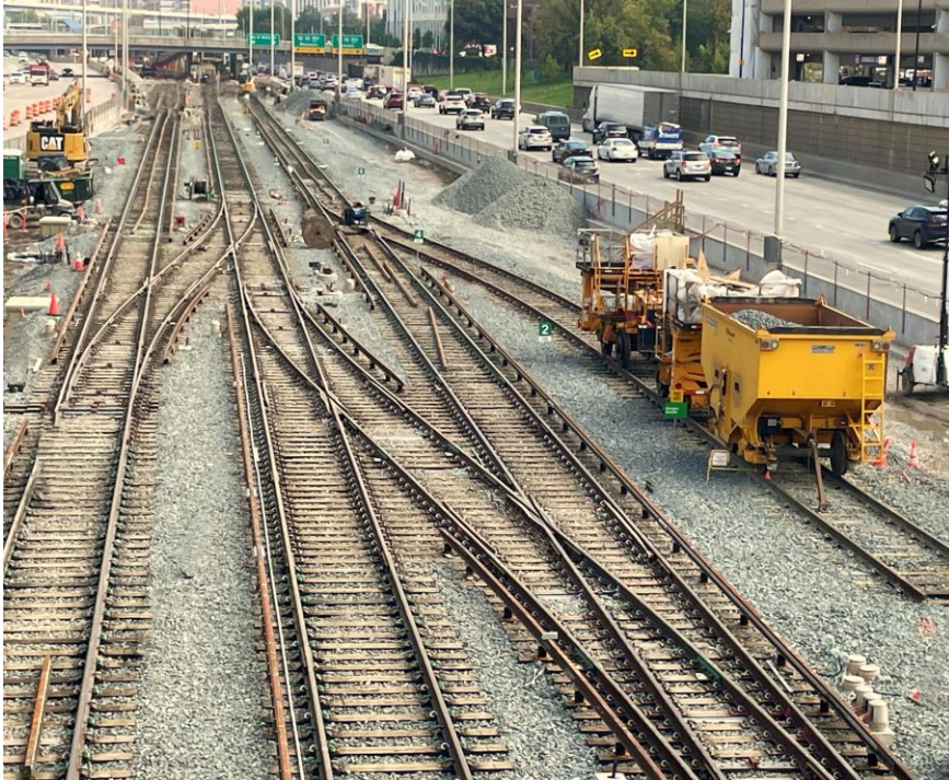
Morgan Middle Special Trackwork
