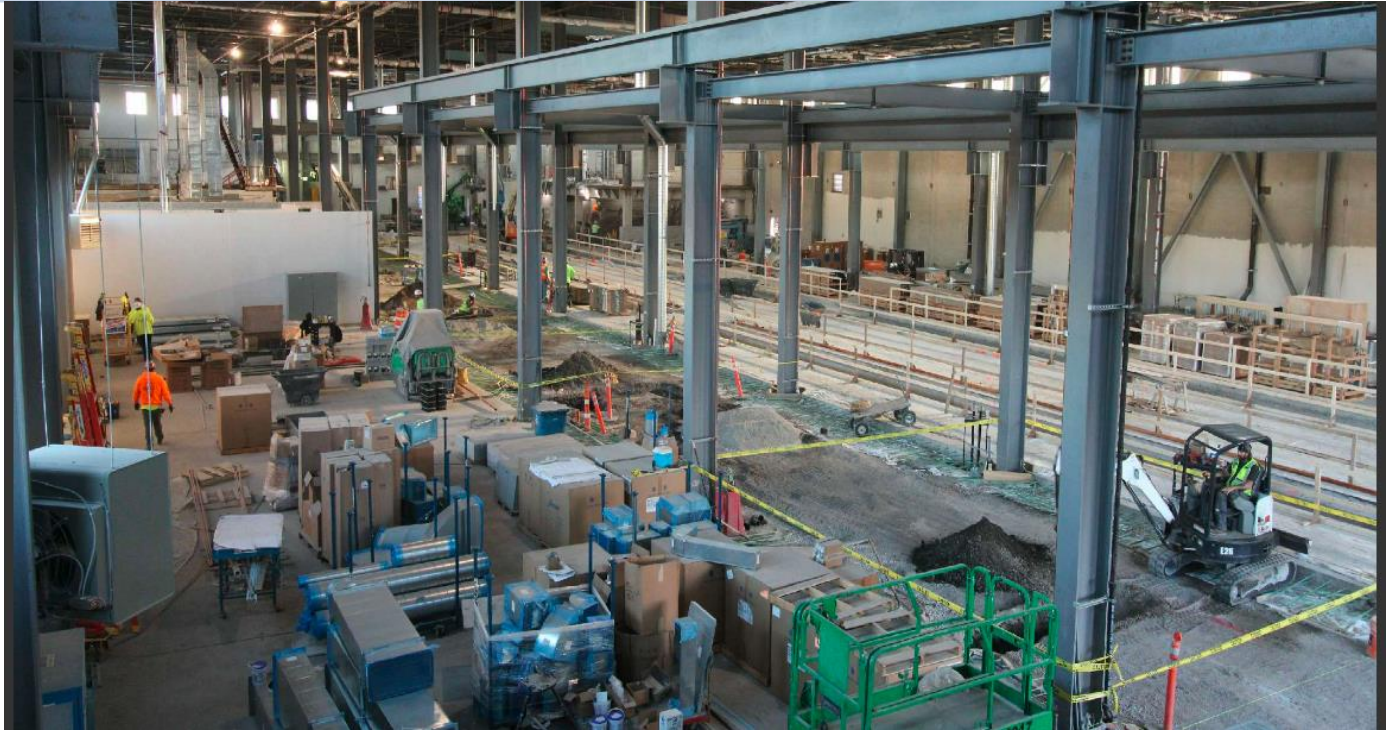
Building Interior – Looking Northeast
