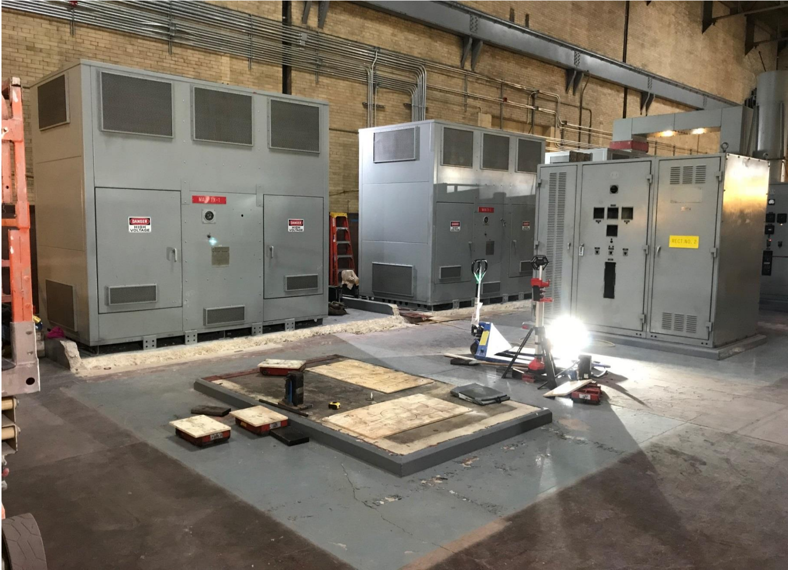
Illinois Substation Demolition of Traction Power Equipment
