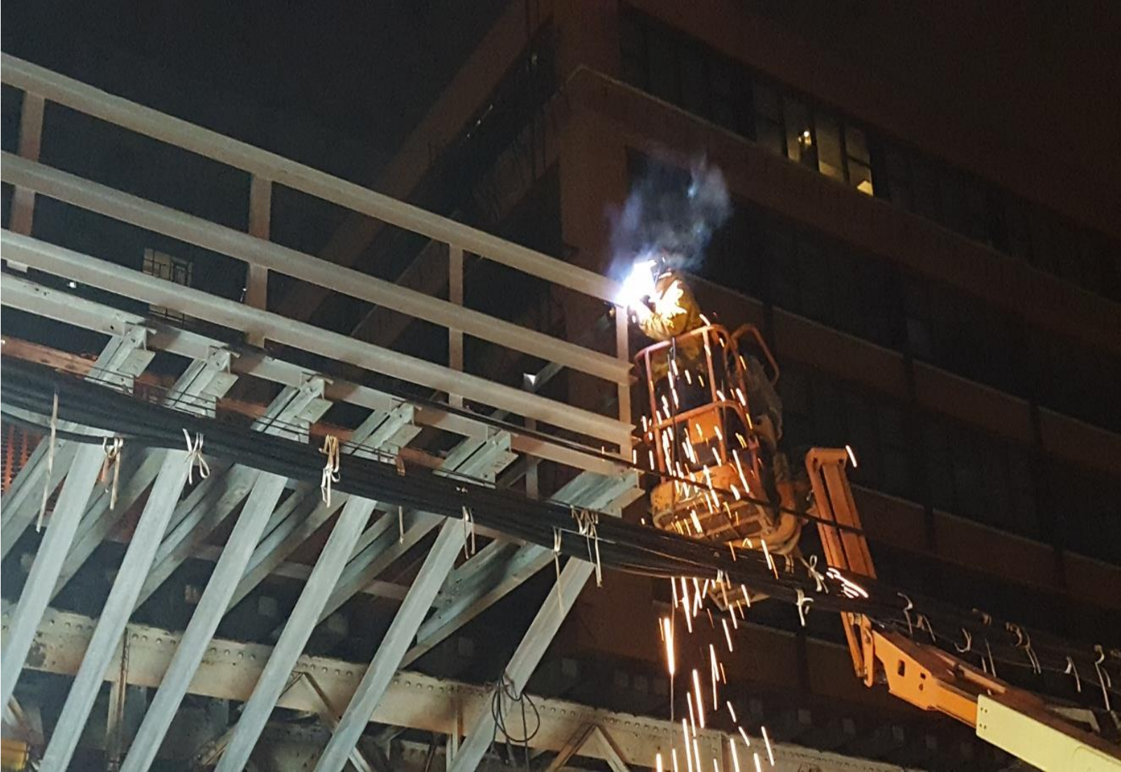
Welding Platform Handrail at Huron St.
