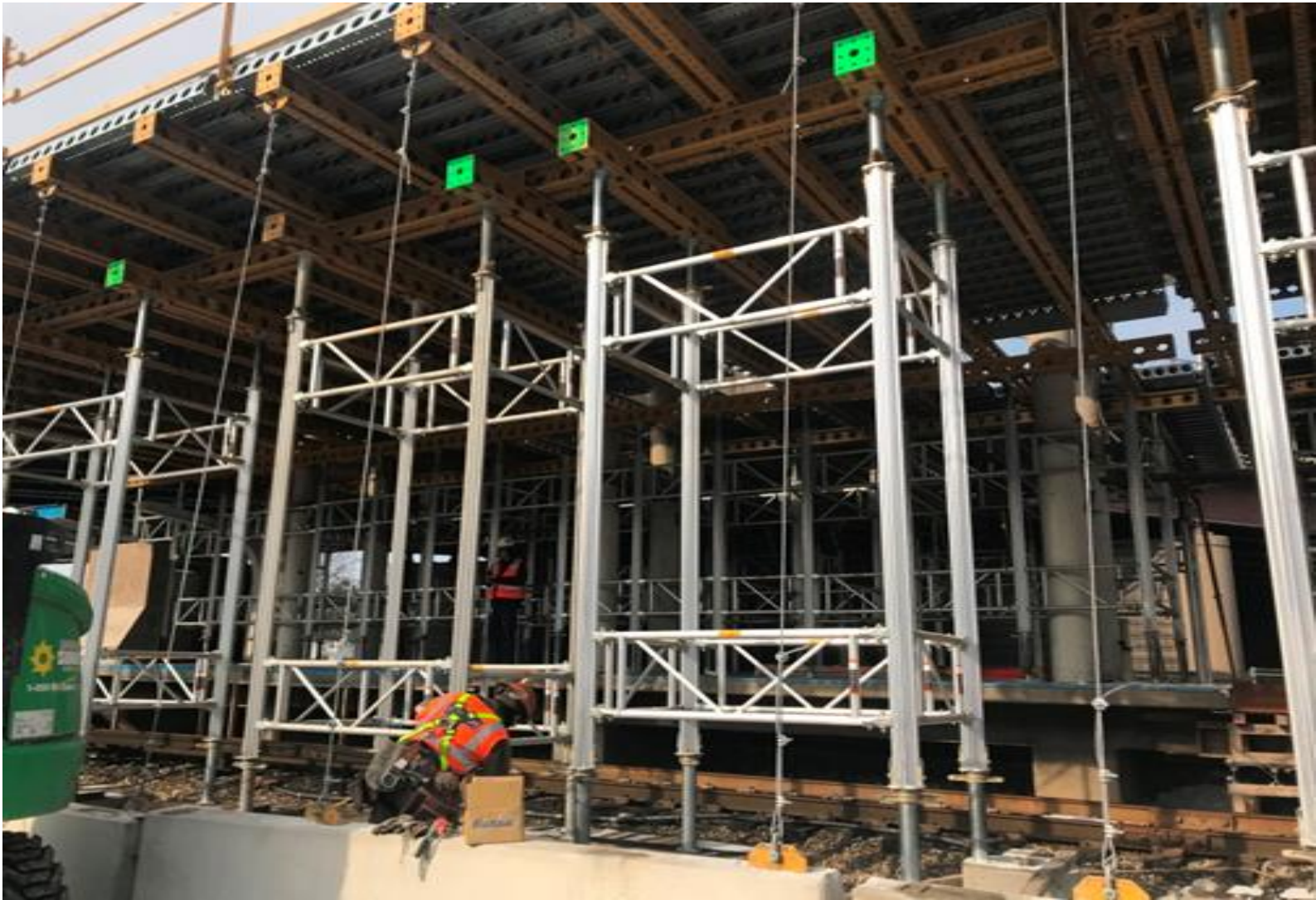
Ogden Stationhouse – Temporary Shoring Installation
