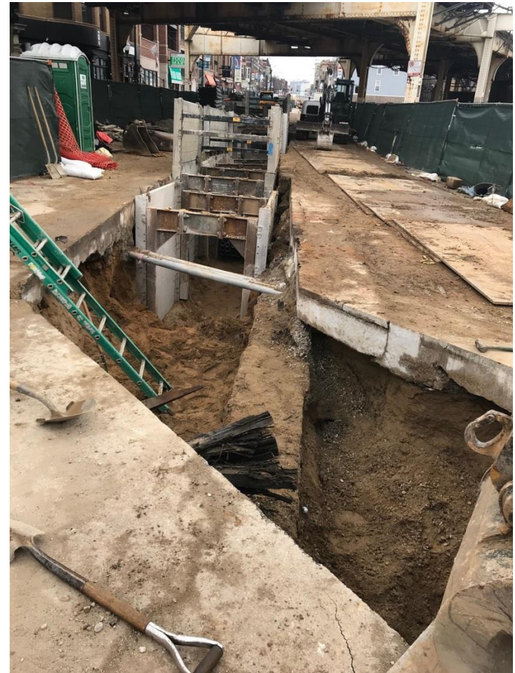
Gas main installation by Peoples Gas contractor (left) and AT&T trench south side of Roscoe (right) on Clark Street
