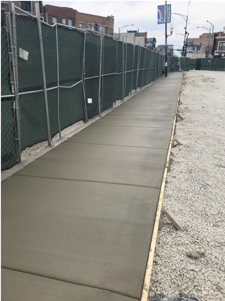
Parcel 14,15 and 16 sidewalk and fencing
