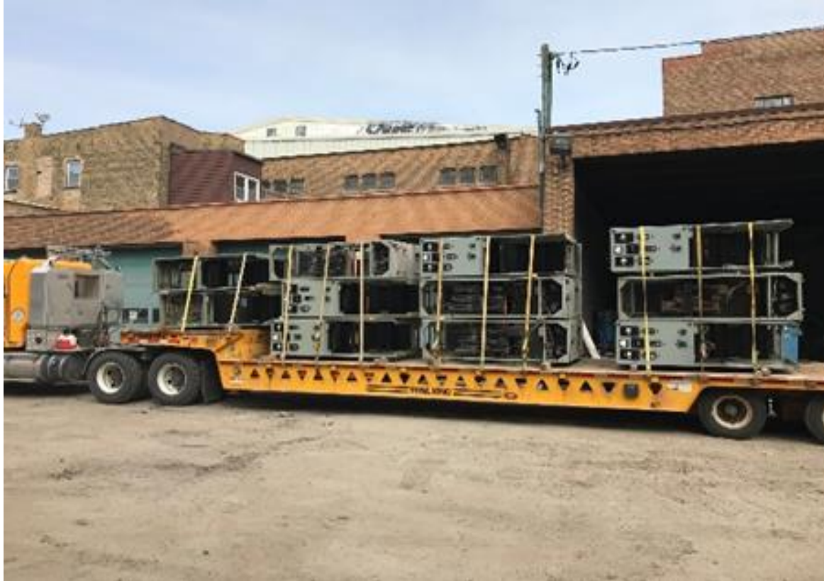
Old Equipment Removal
