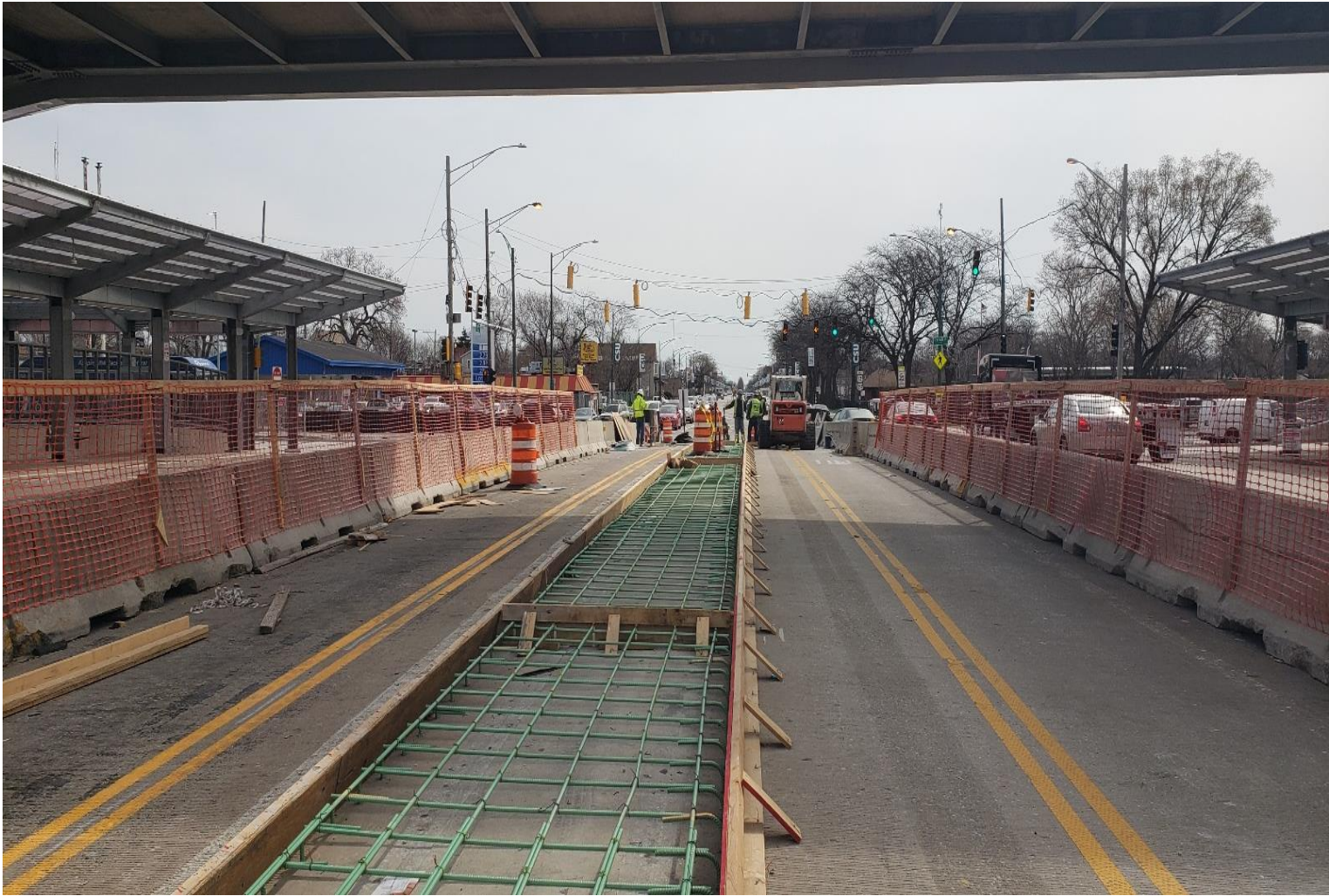
95 th Bridge – Median Preparation
