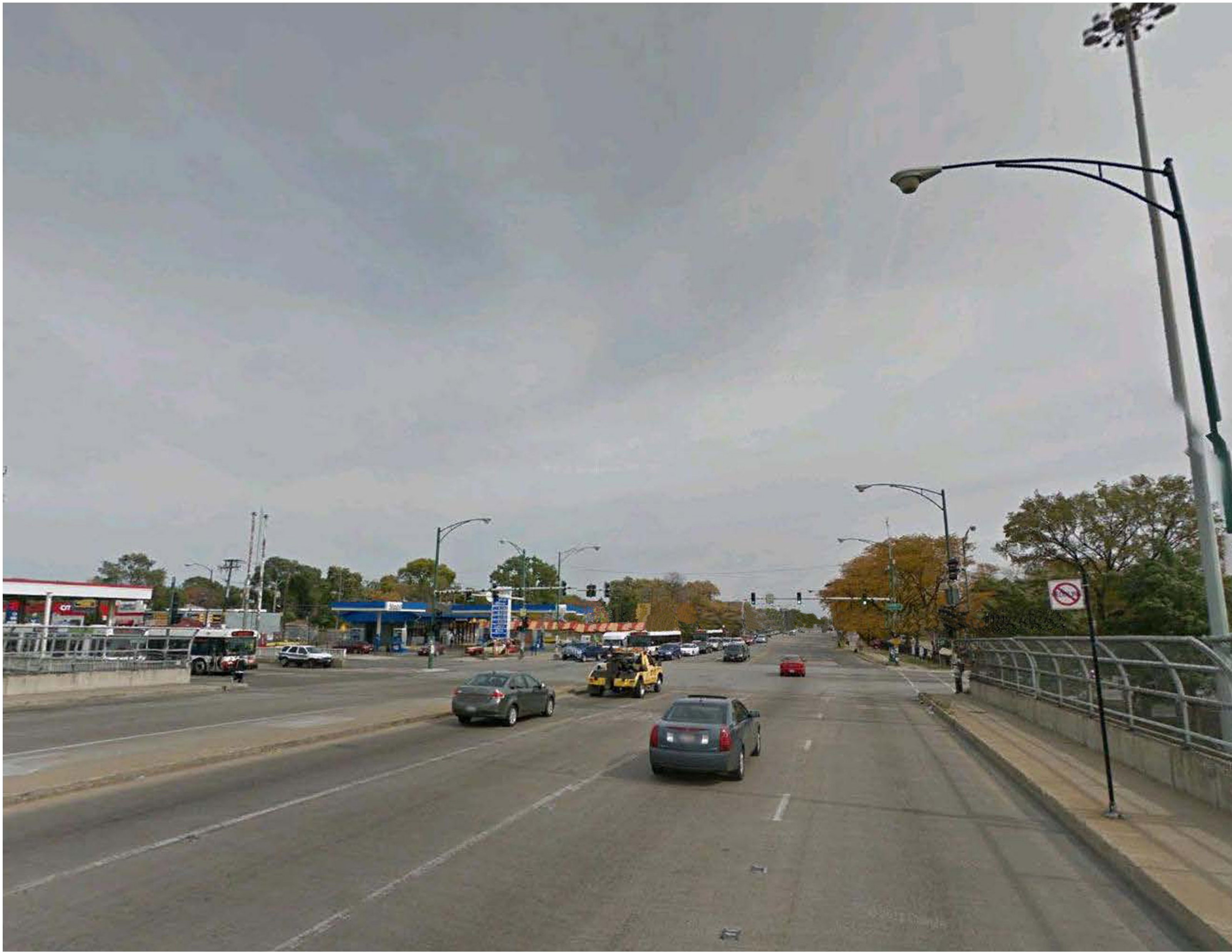
Facing East along 95th Street Bridge
