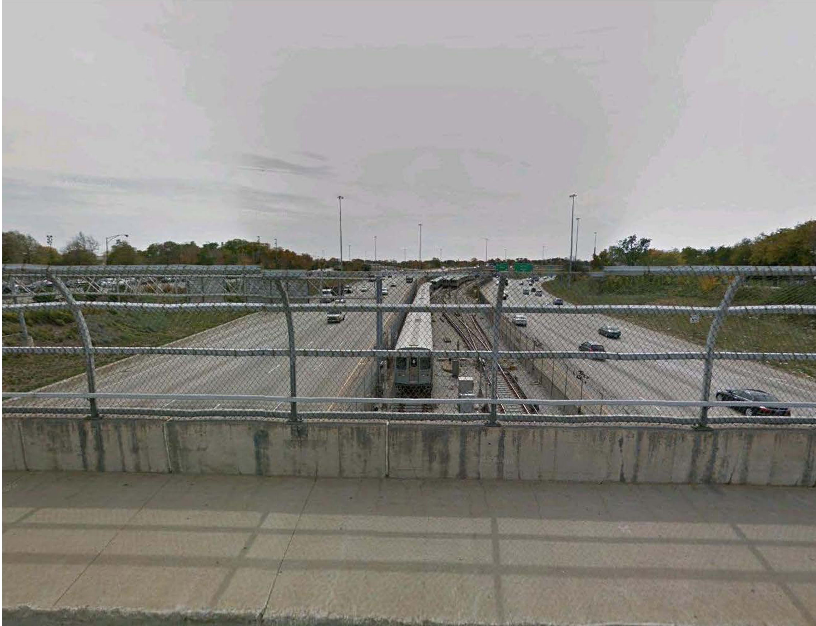
Facing South from 95th Street Bridge
