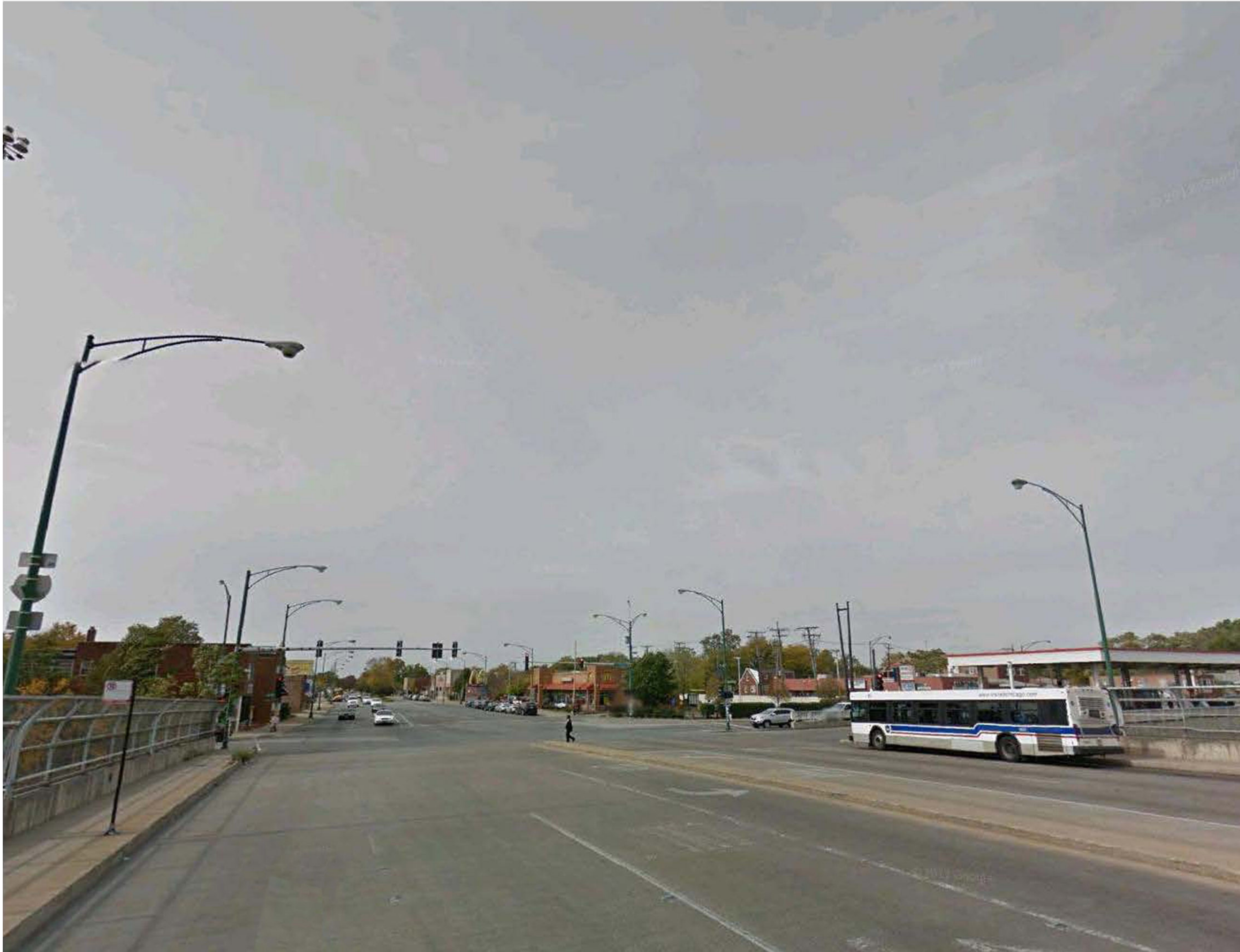
Facing West along 95th Street Bridge
