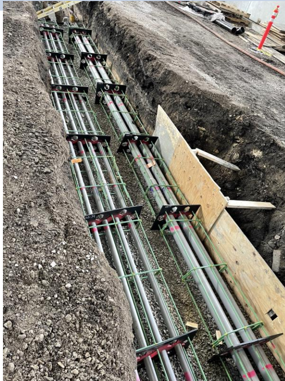
Aldridge – Installing Duck Banks
