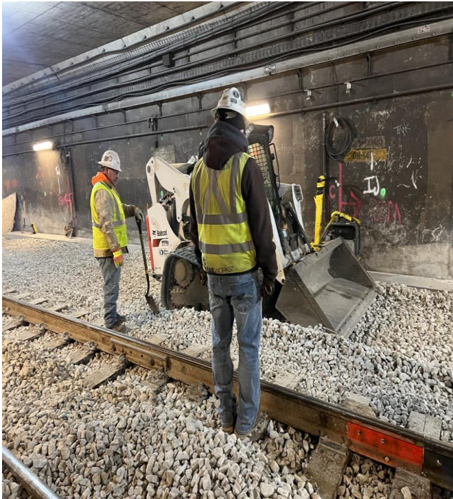
Ballast and Track Installation at Belmont
