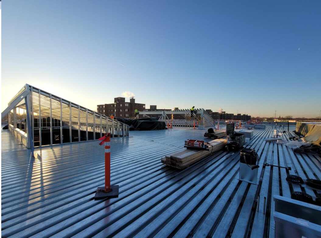
Levy – Clerestory Framing
