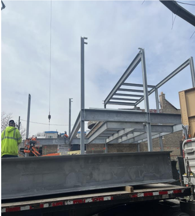
Erecting Structural Steel at Damen
