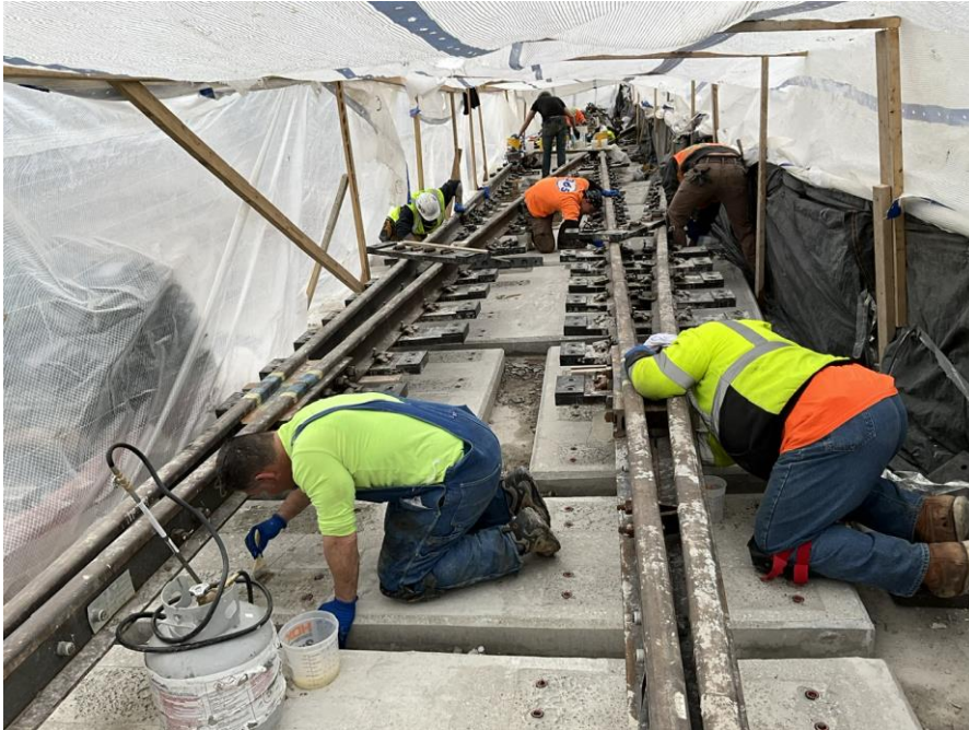
Special Track Work Concrete Patching
