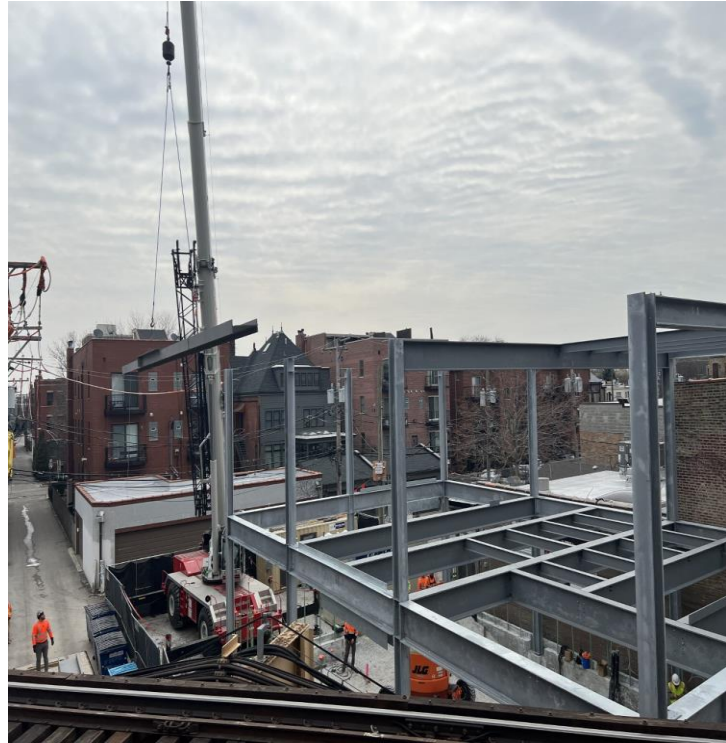
Erecting Structural Steel at Damen
