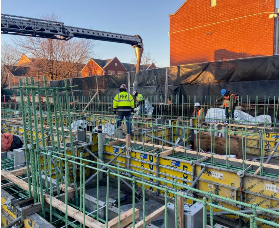
Damen Station Pouring Concrete Grade Beams at Station House (South half)
