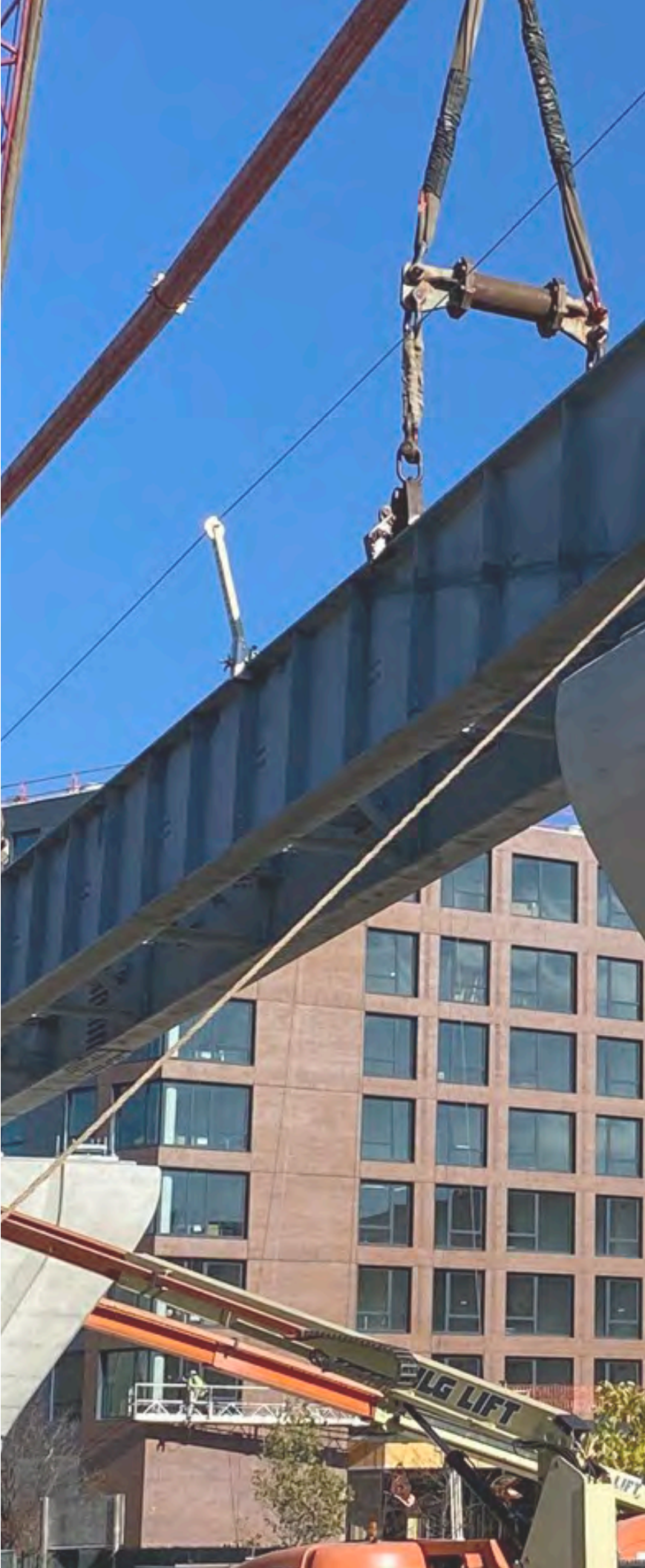
Figure 6-1: CTA Red Purple Modernization, Phase One Brown Line Bypass Construction
