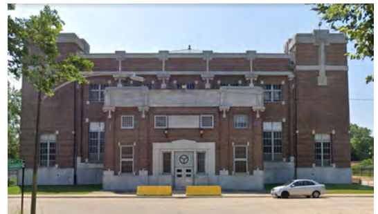
Figure 3-8: Roseland Pumping Station
