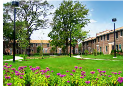
Figure 3-64: Altgeld Gardens Rowhouses Source: Chicago Housing Authority
