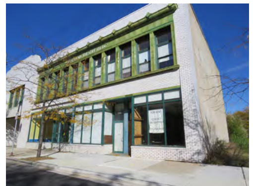
Figure 3-43: Renovated Roseland Theatre Building
