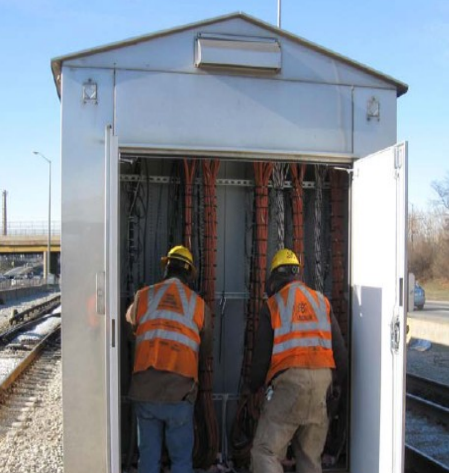
Installation of cable clamps on Blue Line Congress Branch
