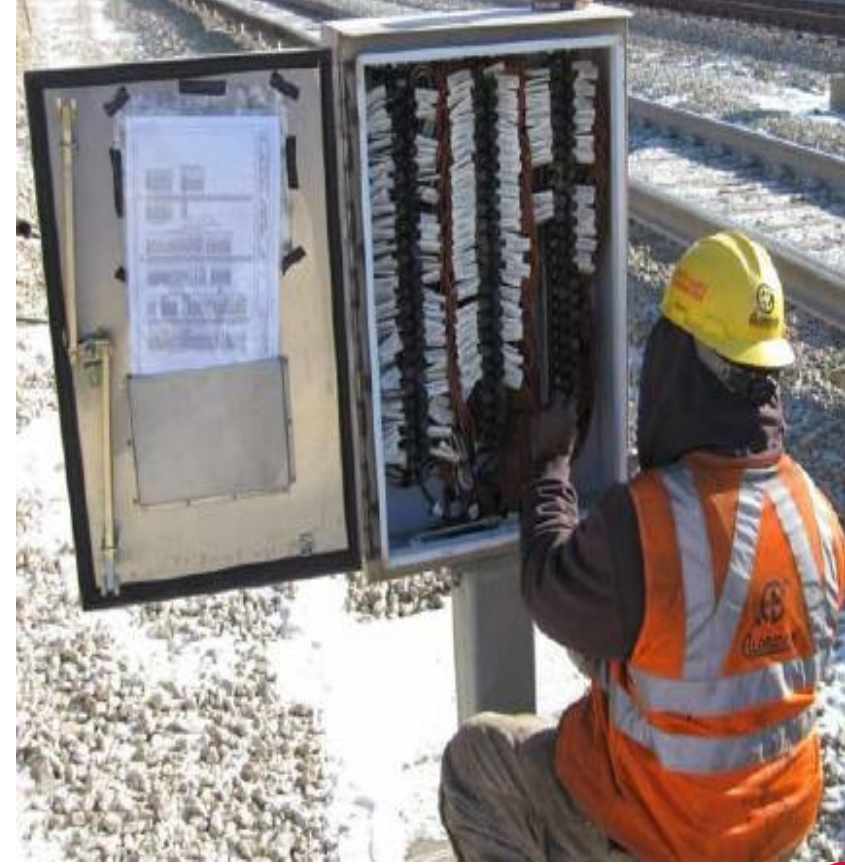
Punchlist work – Junction box work on Blue Line Congress Branch
