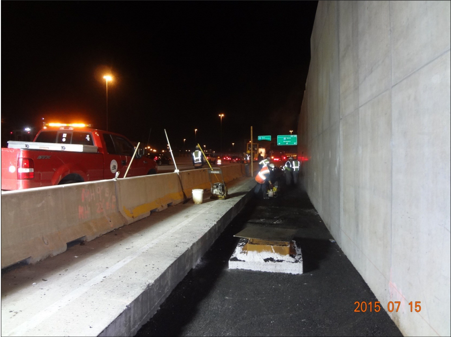
AP2: Shoulder Work on West Side (Wall 1 and Wall 2)
