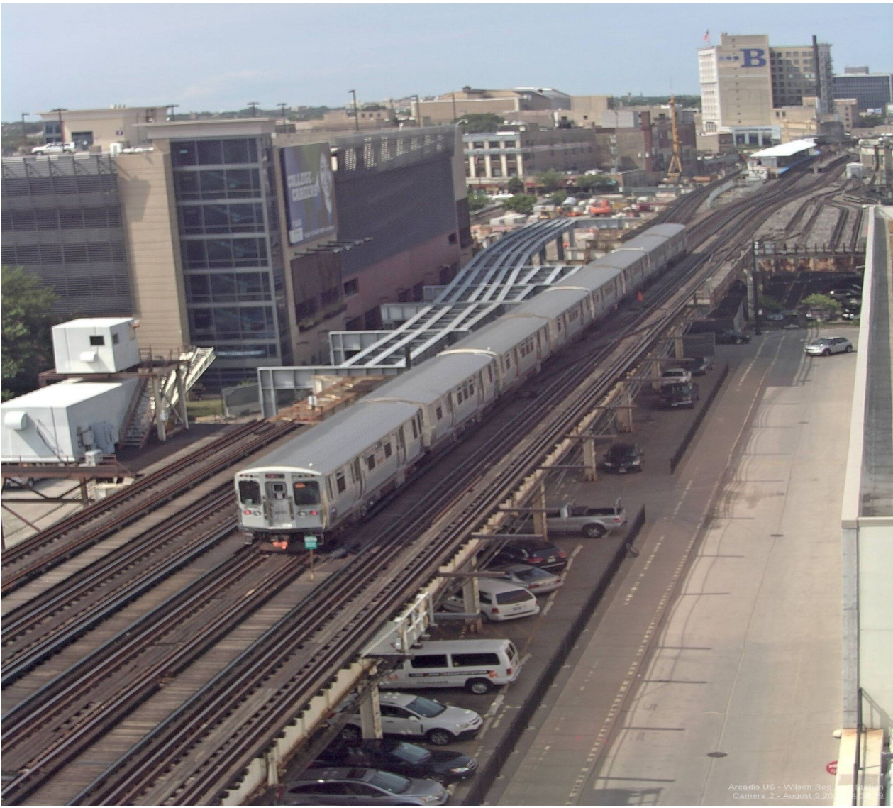
New track 1 steel structure installation – north of Sunnyside
