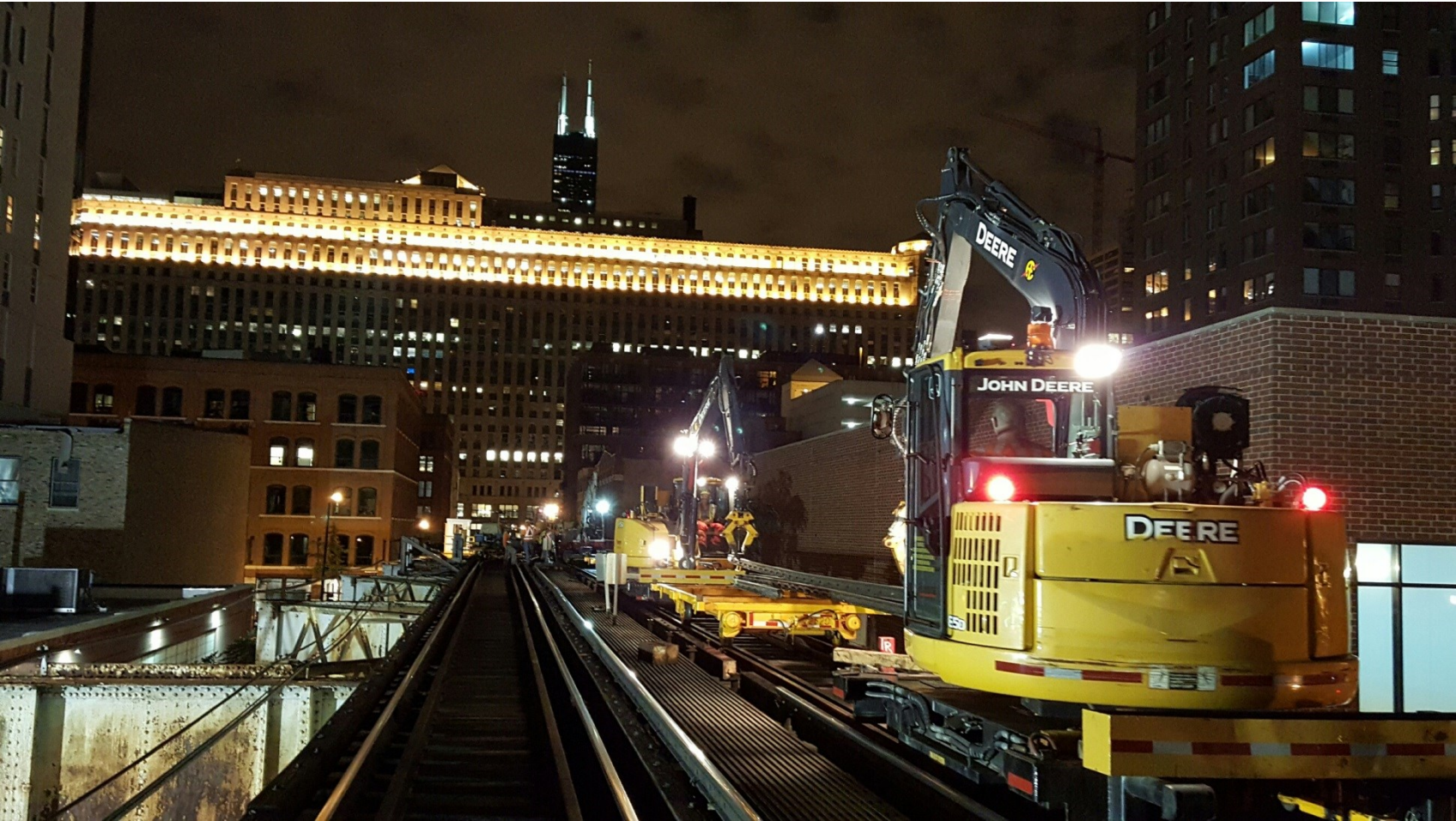
Contractor performing work north of Merchandise Mart
