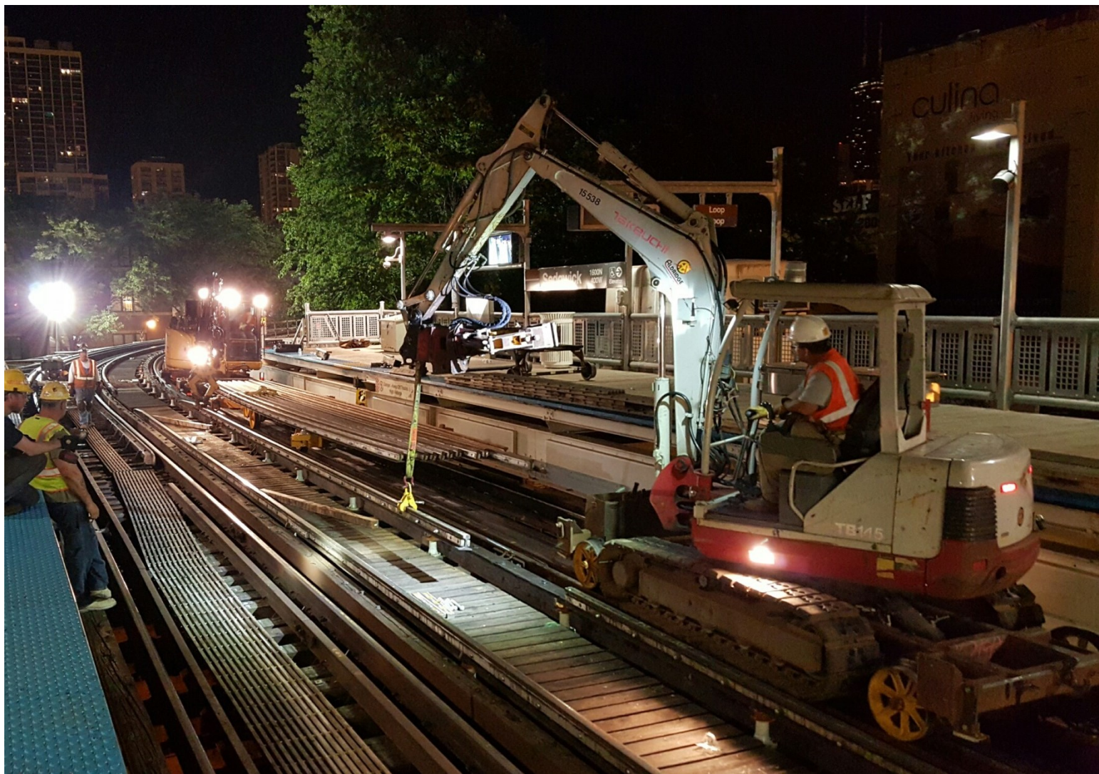
Contractor Installing Third Rail at Sedgwick Station
