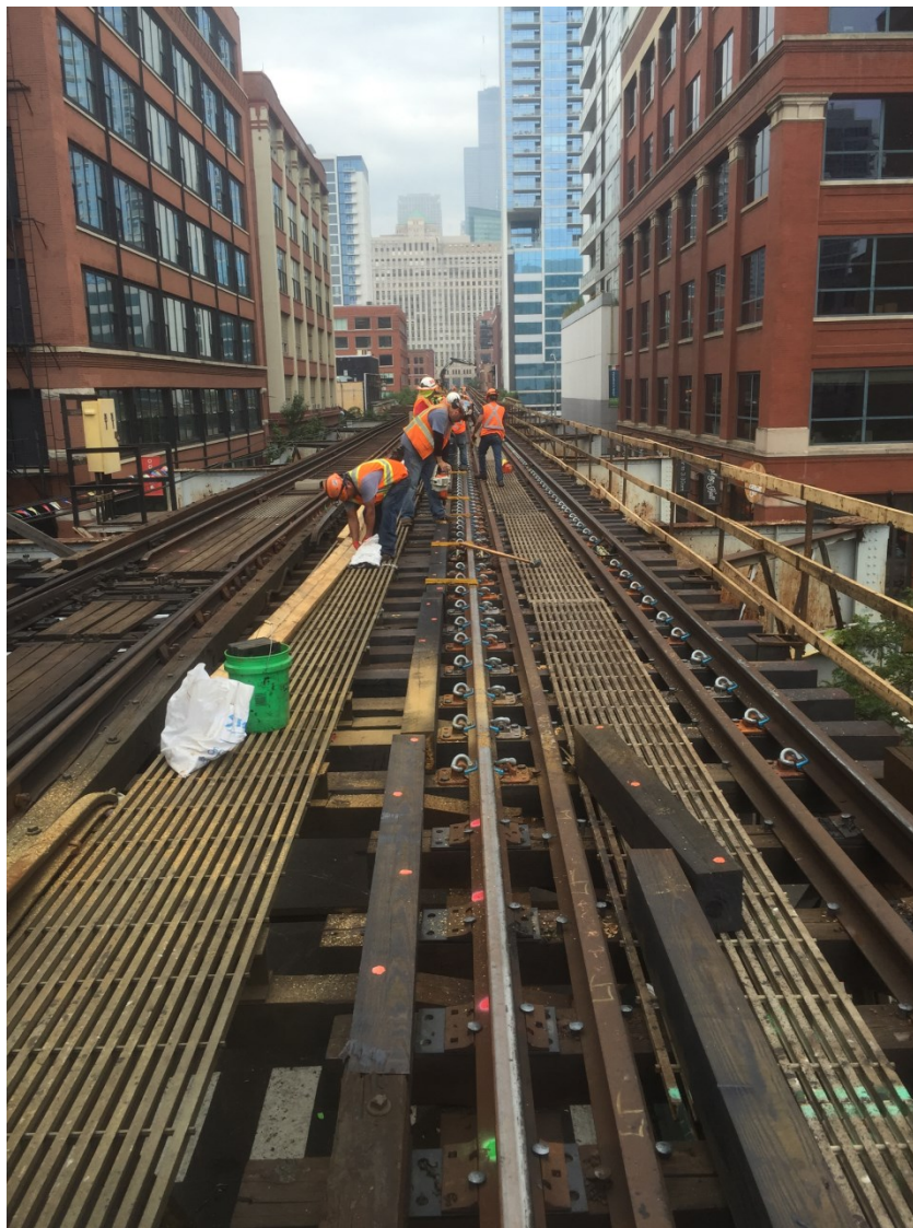
Contractor Installing Track Between Merchandise Mart and Chicago Stations
