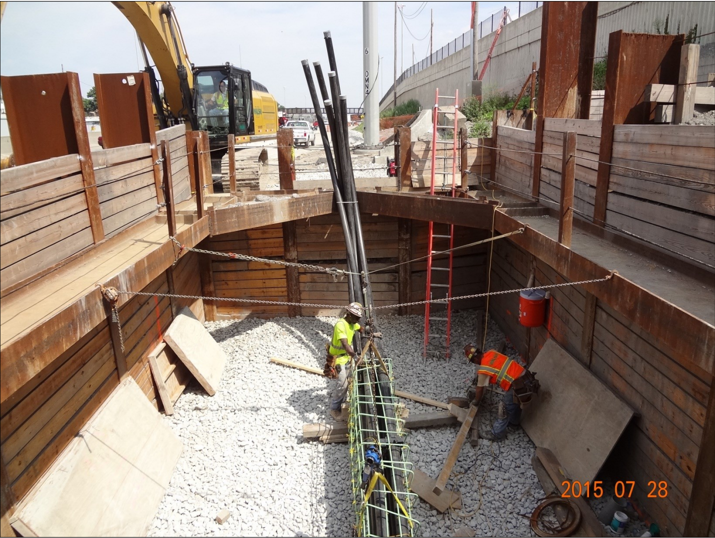
AP2: Ductbank Work on East Side (Wall 6)
