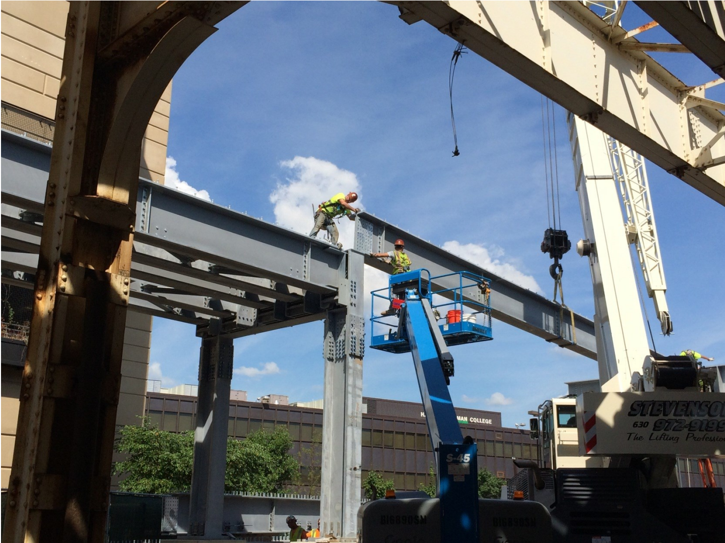
New track 1 steel installation
