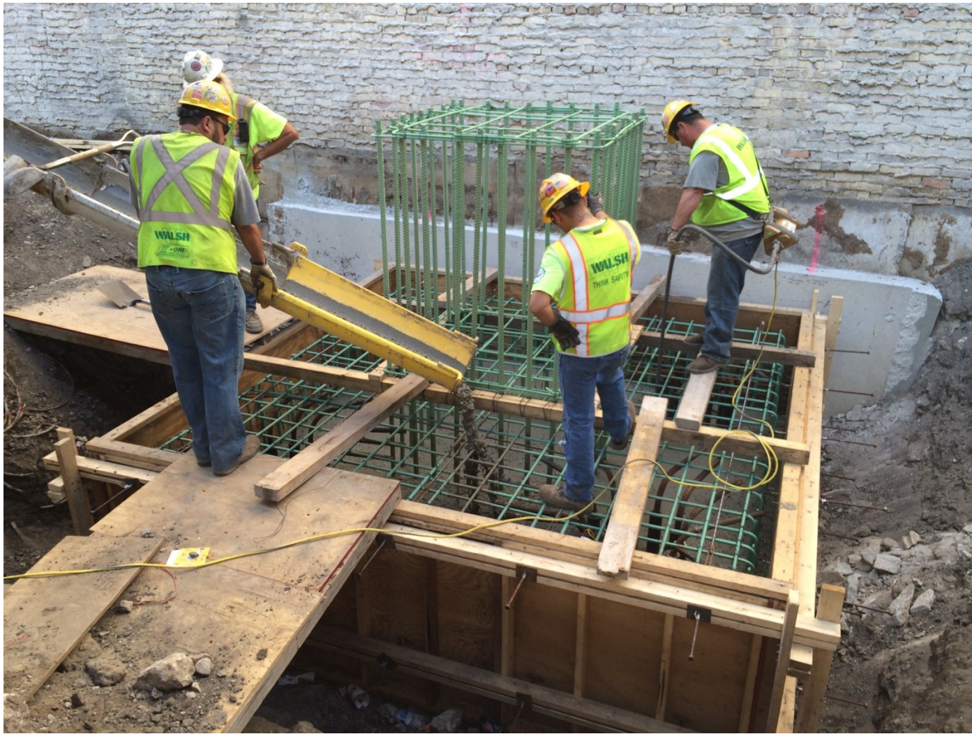
New micropile cap foundation installation – north of Leland
