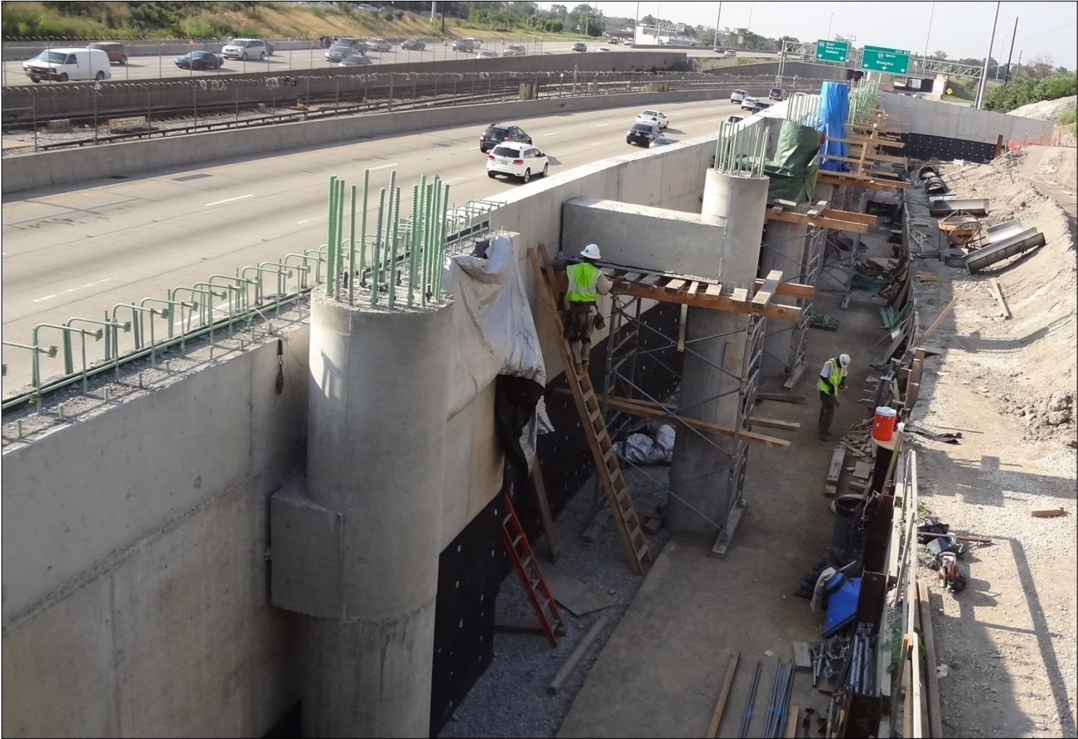
AP2: Column and Strut Concrete Work on Southwest Quadrant (Wall 1)
