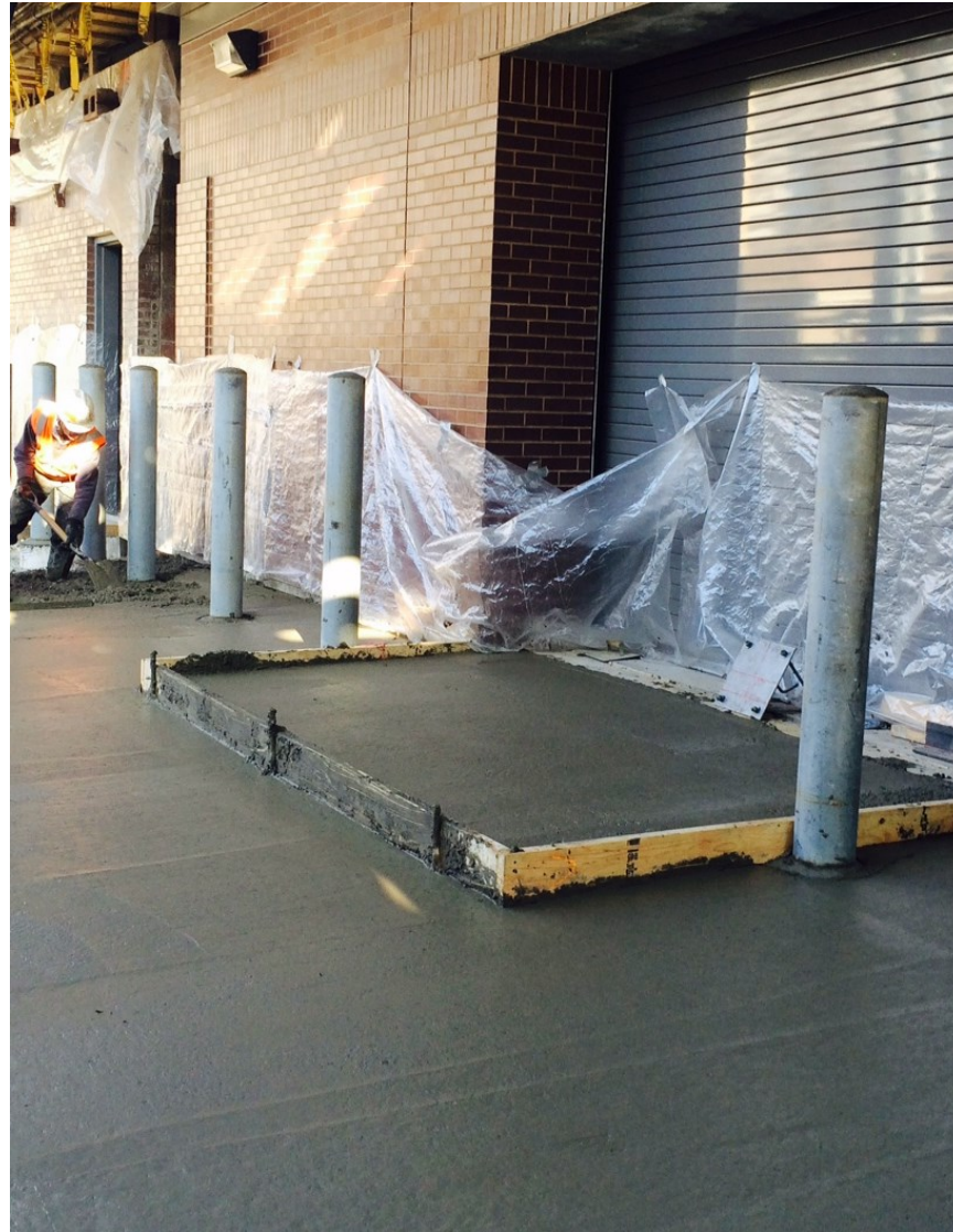
Armitage Substation: Concrete and Bollard Installation (West Face)
